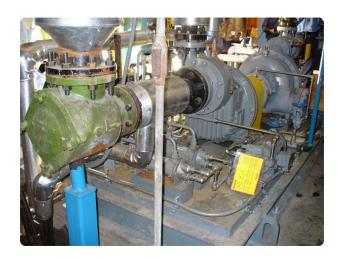
Employers and operators alike are sometimes hesitant to operate existing, or install new steam turbine driven boiler feedwater pumps due to some mis-guided apprehensions and lack of concrete knowledge as to why they can be viable options to electric motor driven feedwater pumps.
